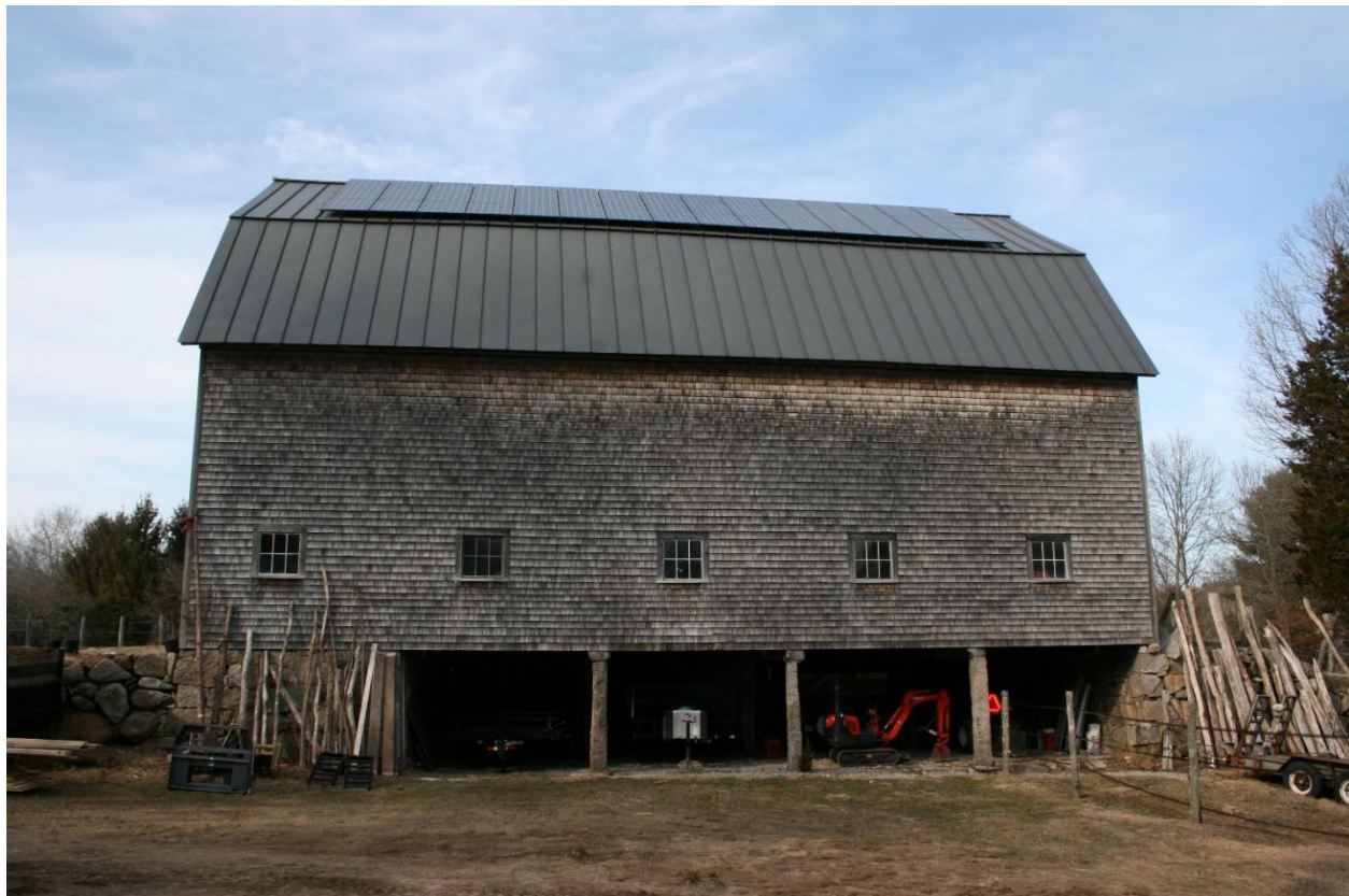
Figure 2: Fluers, Inc. Richmond, RI 8.1kW systems
